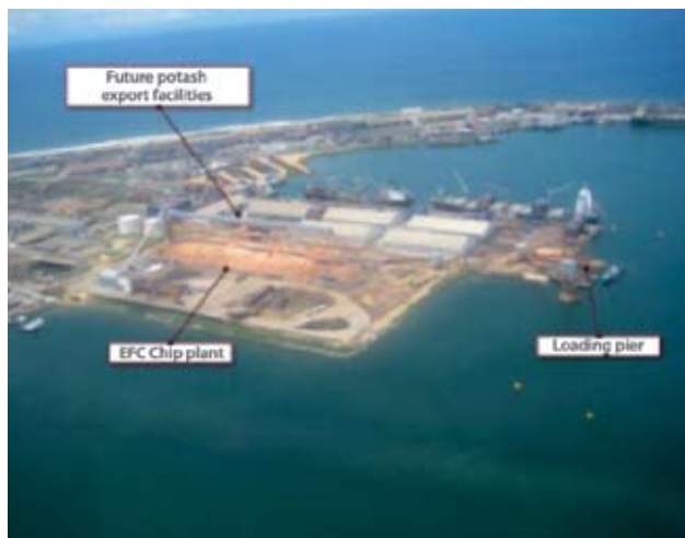
MagIndustries pier within Pointe Noire harbour includes chip mill, loading pier and future potash export terminal.
