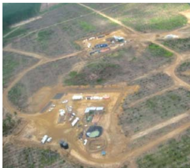
Drilling of solution brine wells at Mengo advancing quickly.
