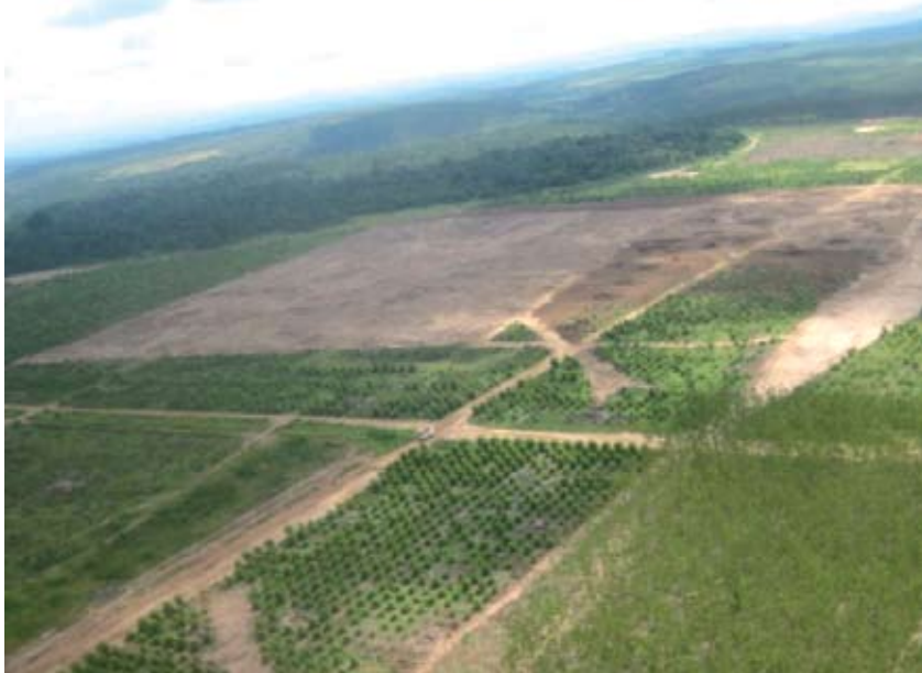
Pre construction ground work for the potash plant.
